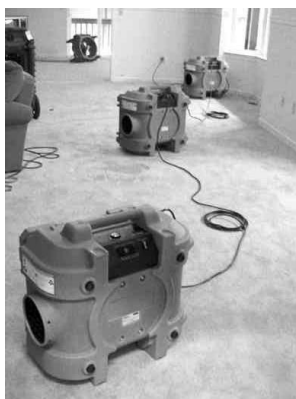
FIGURE 5 Units daisy chained
