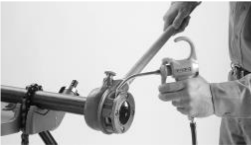
Figure 4 – Applying Thread Cutter Oil
